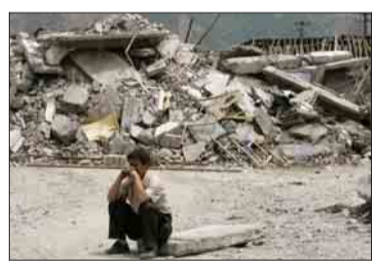
Despair and devastation at a collapsed school building in Wenchuan. Photo: Reuters
